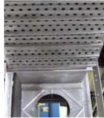
Interior section of system under construction showing upper air supply duct
